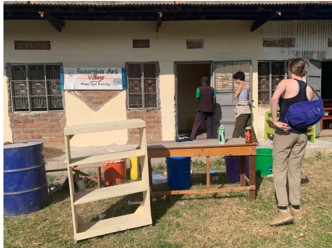
Photo: library renovation and painting in progress
